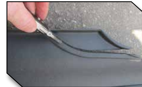
Figure 10 - Trimming Along Rib
